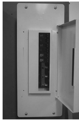
Step #3 Install New HFLCI
