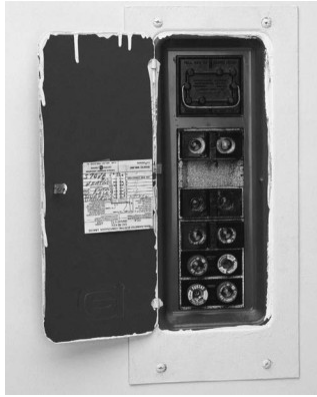
Step #1 Identify Box Dimensions and Catalogue Number
